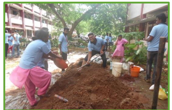
Volunteers working at the Civil Station Compound
