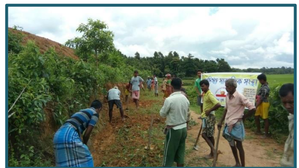
Volunteers building the road in Udaipur, Tripura
